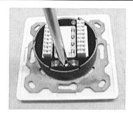
Take out the cover. Loosen the M-shape cable holder and take it up.
